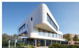
Office and administration buildings
