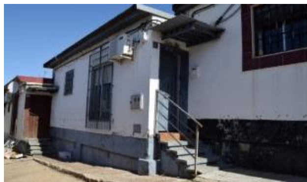
Original state of the building
