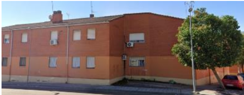
Original state of the building
