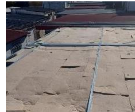
Kenaf insulation on the roof
