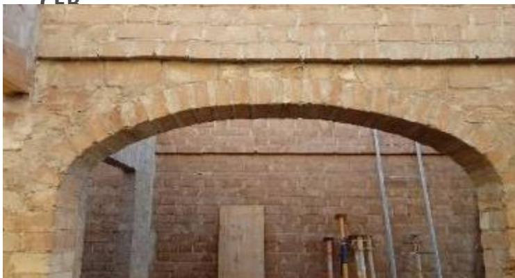
Execution of walls and arches with CEB
