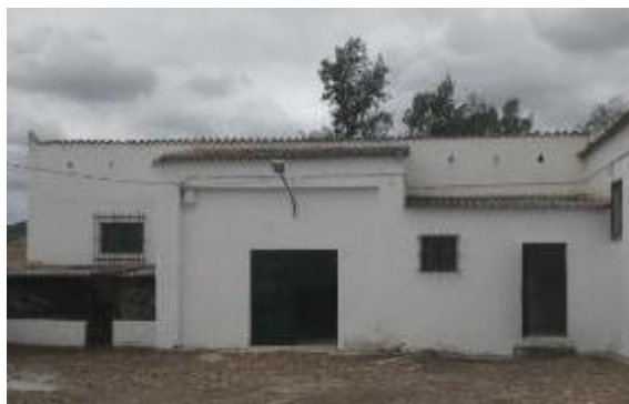
Original state of the building
