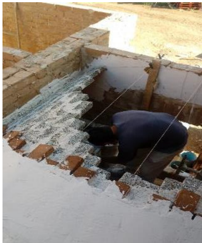
Execution of vault with wood wool board and CEB
