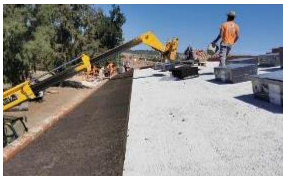
Cork insulation on the roof
