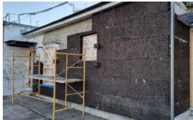
Cork insulation on the façade
