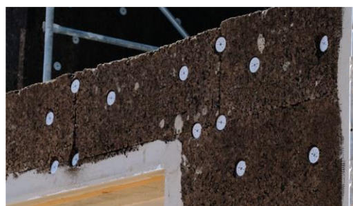
Cork insulation ( \lambda=0,040 - 0,045 W/mk)
