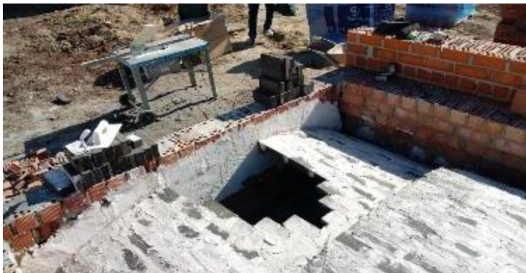
Execution of vault with foam glass and CEB
