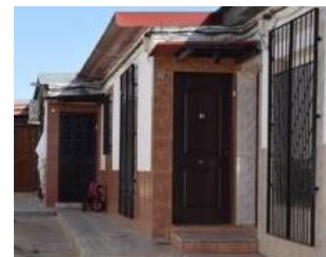
Original state of the building
