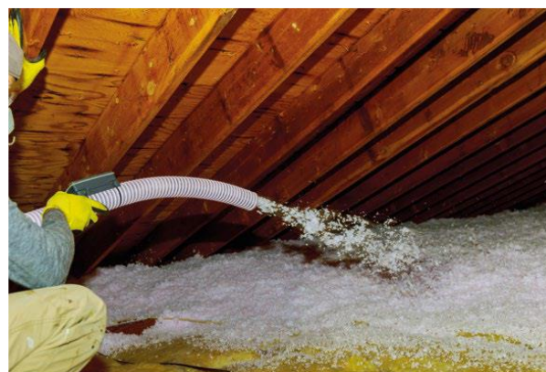
Cellulose insulation ( \lambda=0,022 - 0,035 W/mk)
