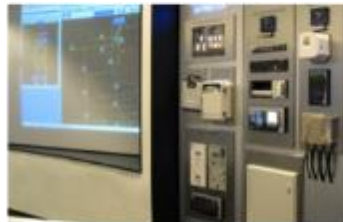
Performance monitoring & display. Building as a pedagogical tool
